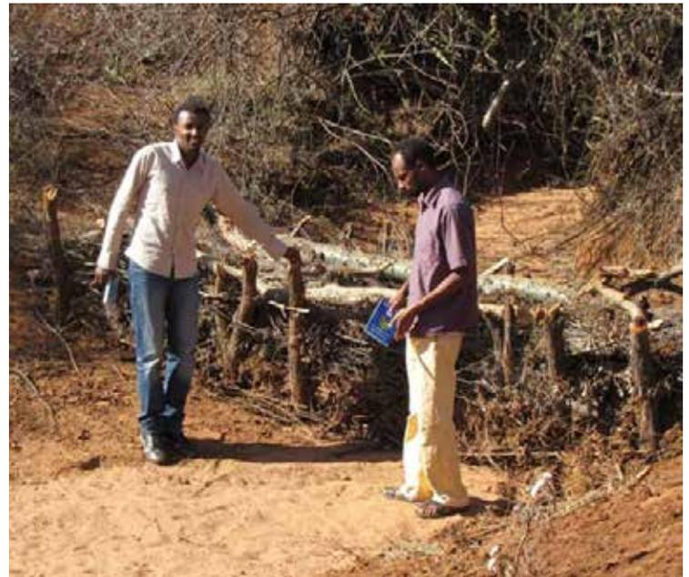
*A large sieve-dam structure in a gully on the central Borana Plateau. (Photo credit: Brien E. Norton)*
