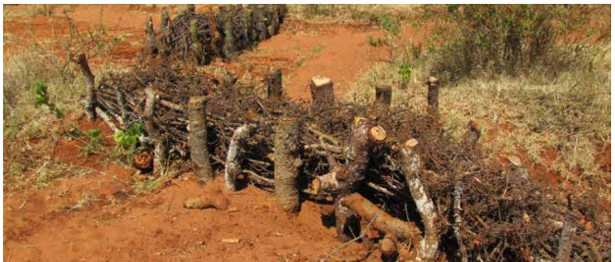
*A pair of sieve structures at the confluence of 2 secondary gullies in the Dikale enclosure. The basic design consists of two rows of tree stumps sunk into the gully floor and packed with acacia branches. Some excavation has occurred in sand at the base of the sieve near the camera due to animal activity. (Photo credit: Brien E. Norton).*
