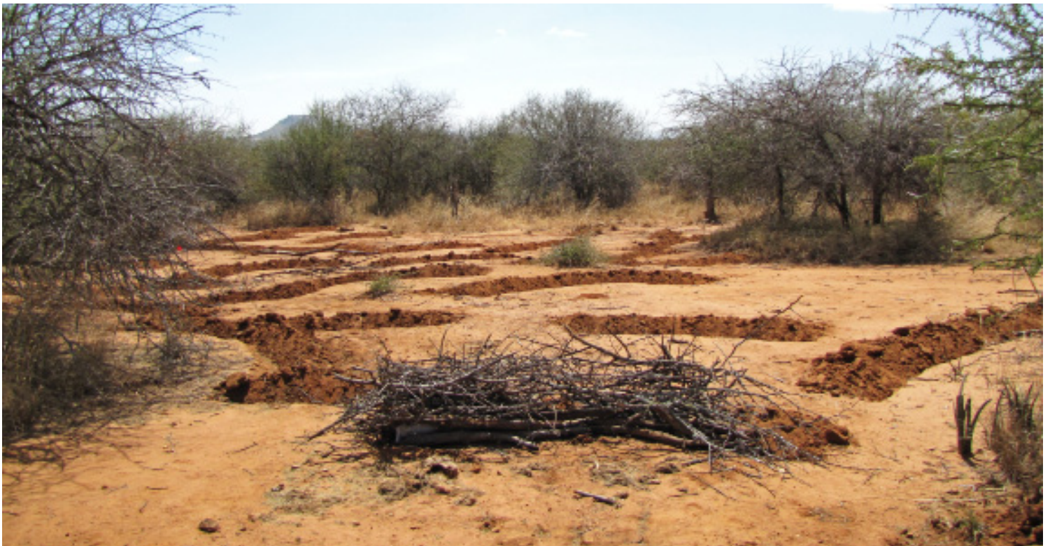
Scaling up -- installing barriers over a large area (about 10 hectares) – a mix of plastic mesh sack barriers and trenches. (Photo by Corinna Riginos)
